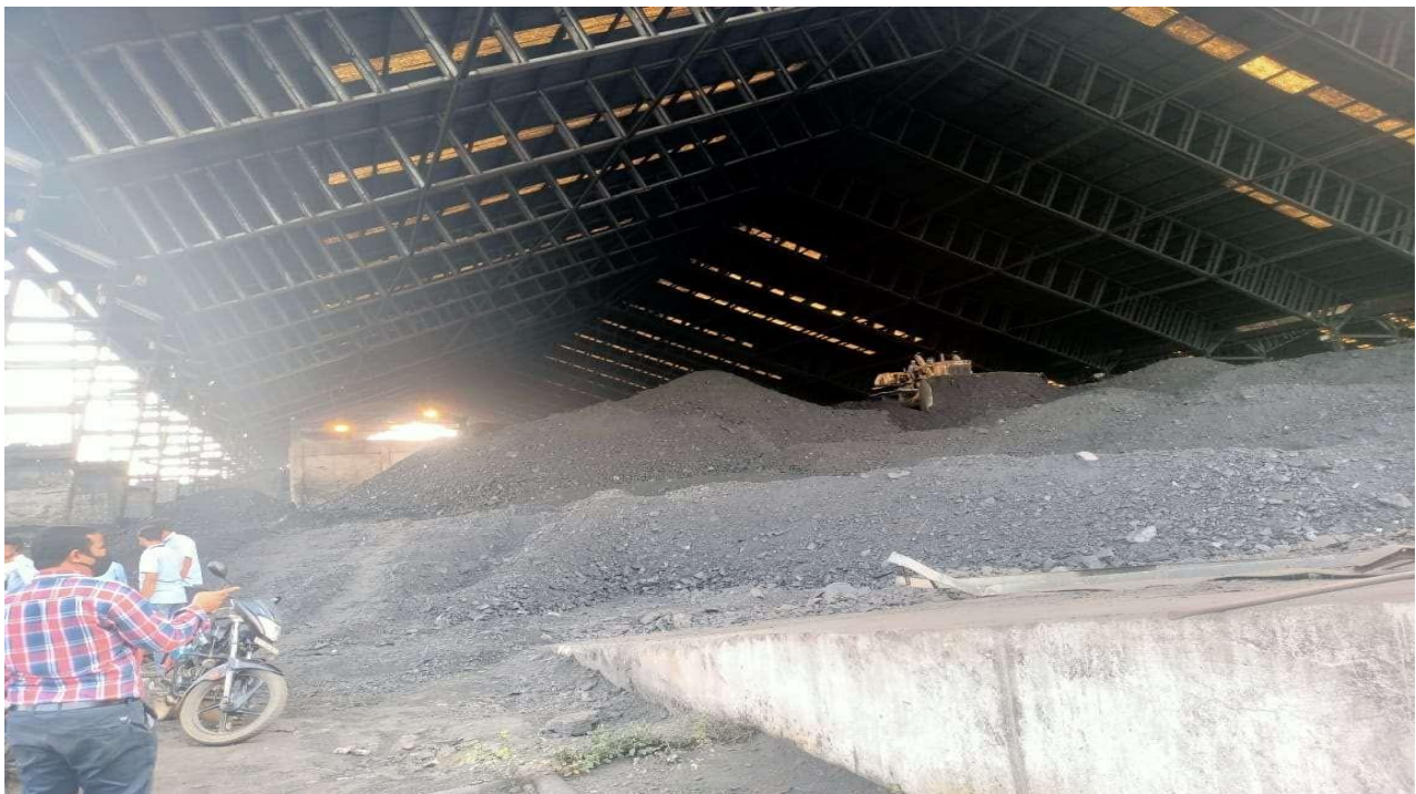
Fig. Coal handling plant
